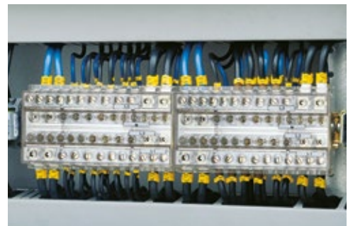
Examples of the use of Z50-DP12-160 and Z35-DP14B-125 type distribution blocks within electrical switchboards
